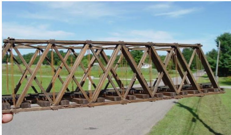
Howe truss Bridge
