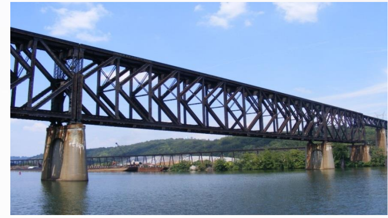
K- truss Bridge
