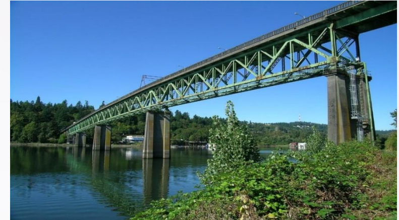
Baltimore truss Bridge
