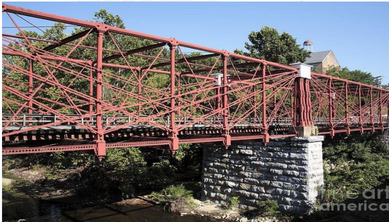
Bollman truss Bridge
