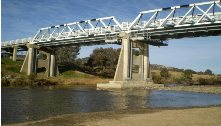
Allan truss Bridge
