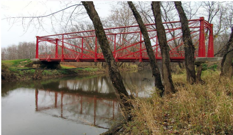
Fink truss Bridge
