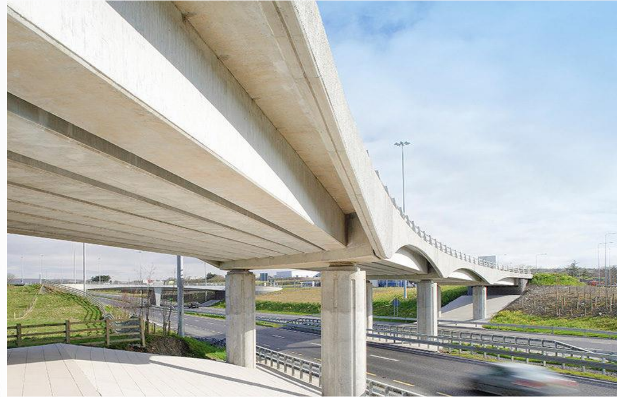
Precast Pretensioned Prestressed Concrete Bridge Simply-Supported Beam
