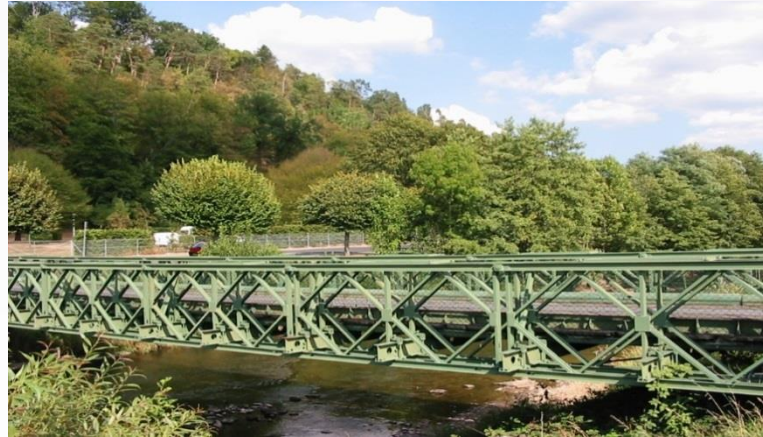
Bailey truss Bridge
