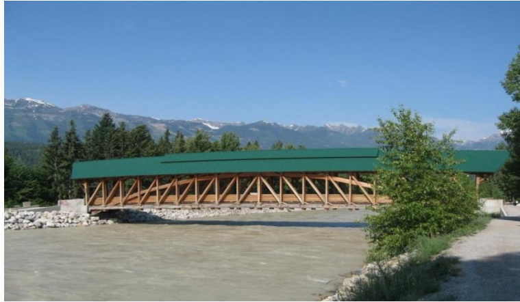
Burr arch truss Bridge
