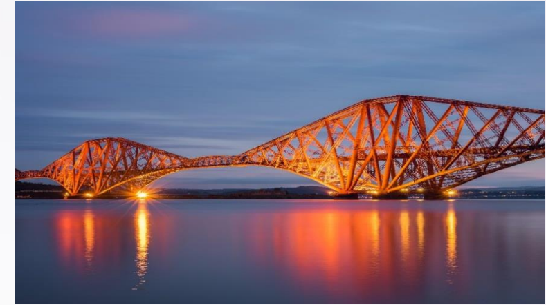
Cantilever truss Bridge
