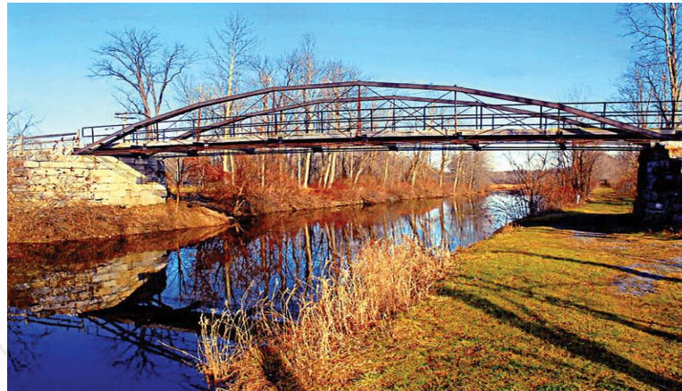
Bowstring truss Bridge
