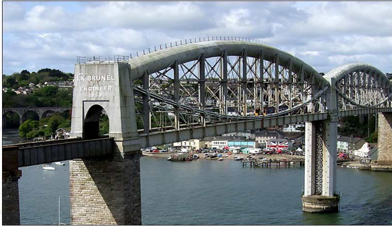
Brunel truss Bridge
