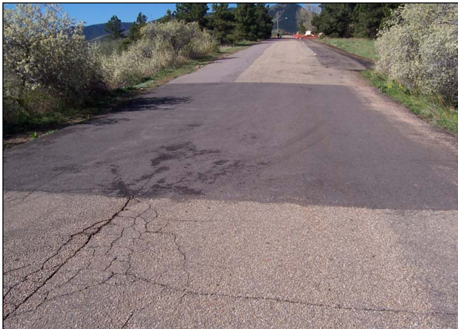
FIGURE 17: Full and Partial-Width Road Patching
