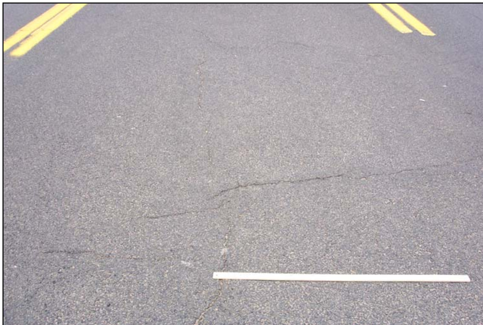
FIGURE 6: Low Severity Alligator Cracking with Few or No Interconnecting Cracks
